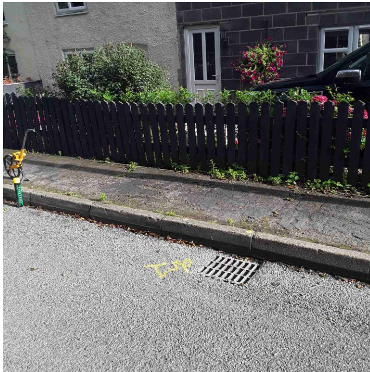
Photo from tablet device on site where flooding was reported on 17 August and a job was issued on 19 August to carry out jetting, investigation and any required civil works for repairs from gully to outfall to two gulleys. Note that water had subsided but officer determined there is still an issue.
